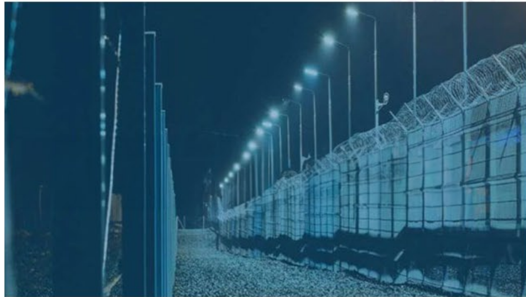
Perimeter Security & Intrusion Detection System
